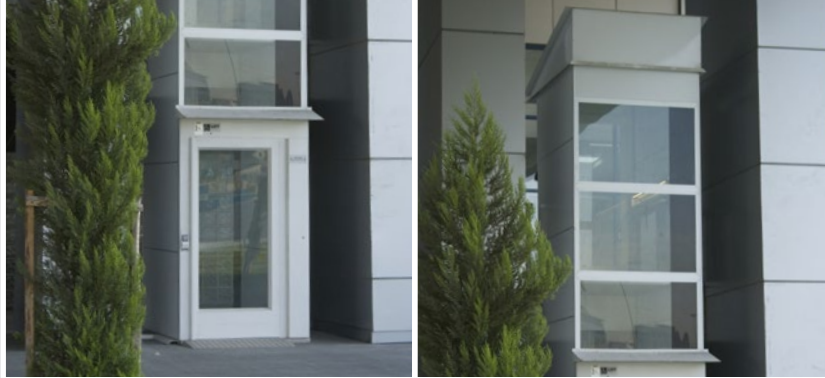
Vertical Wellless Elevator /// İstanbul
