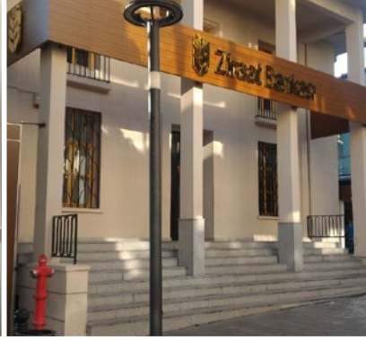
Platform Lift /// Marmaris
